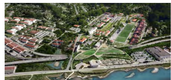
PRESIDIO TUNNEL San Francisco
