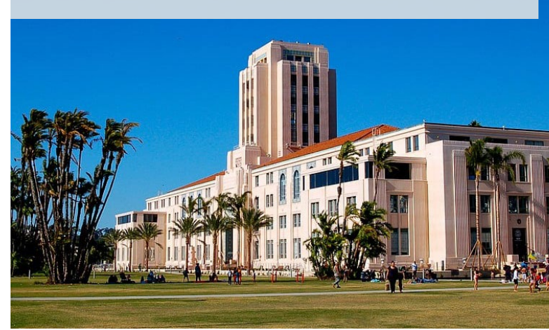
SAN DIEGO COUNTY ADMINISTRATION BUILDING
